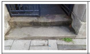
The alleyway is accessed via 2 old uneven steps measuring roughly 9cm & 15cm high with a depth of 38cm.
