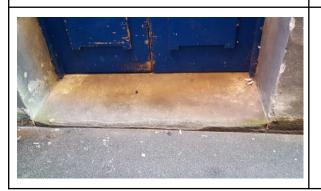
To access the door there is a step up which is uneven and worn, it is approximately 6cm high.
