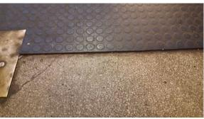
47cm from the mat is a level change to rubber flooring, the rubber flooring sits less than 1cm above the level of the stone floor.
